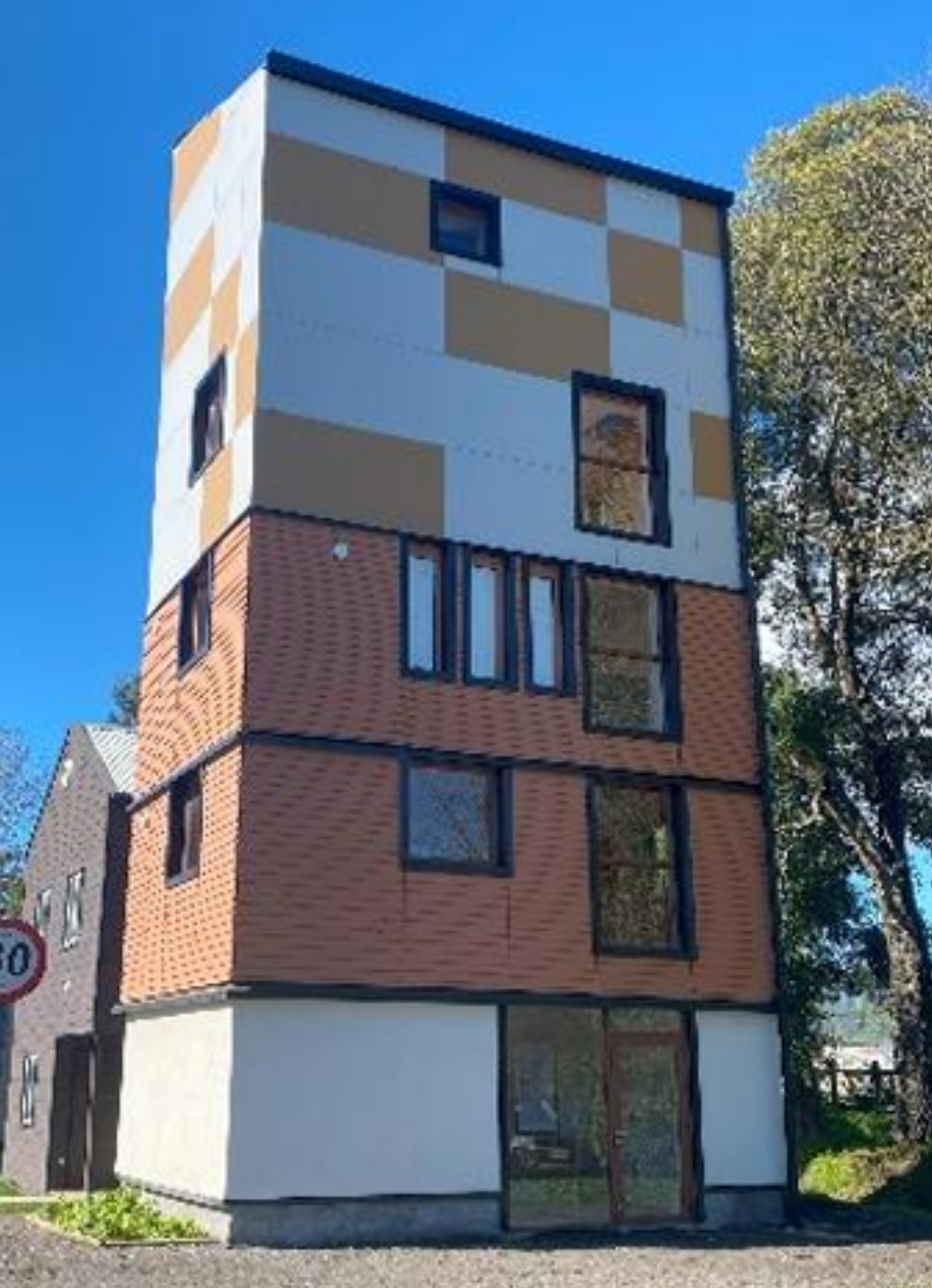
Vista exterior torre Pymelab
