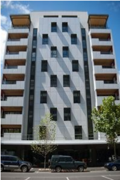
Lend Lease's Forte apartment complex in Melbourne's Victoria Harbour 10 pisos, 32 m, CLT
