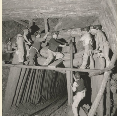
4 INTERIOR MINA DE CARBON
