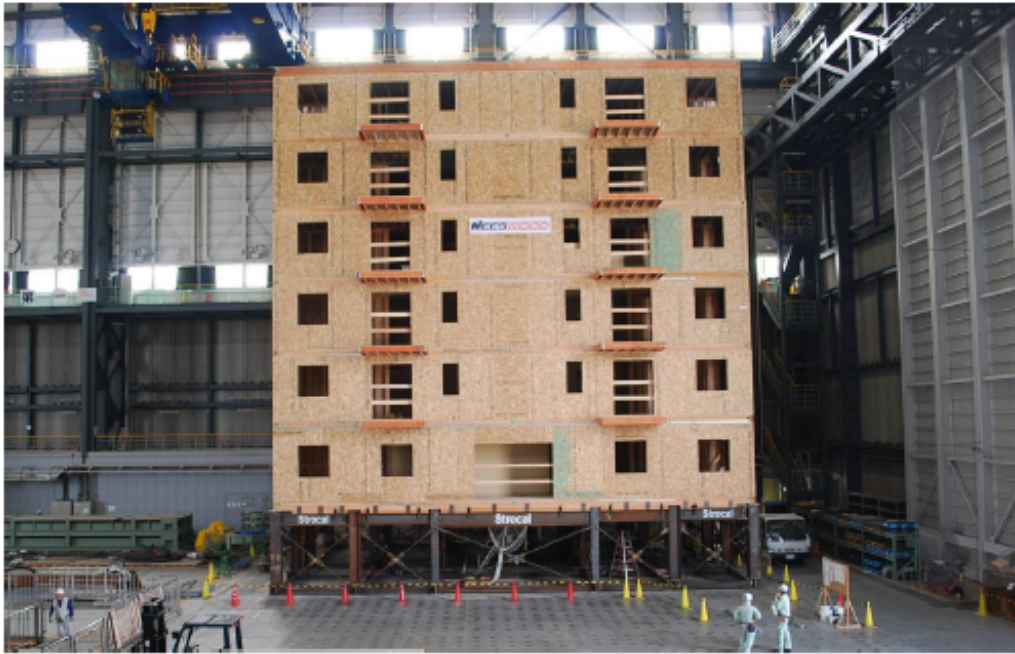
Figure 2.6: Completed Capstone test building at the construction site inside the E-Defense laboratory
